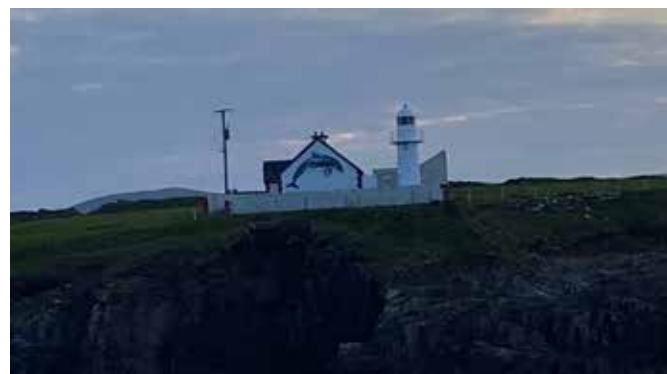
Entrance to Dingle Harbour
